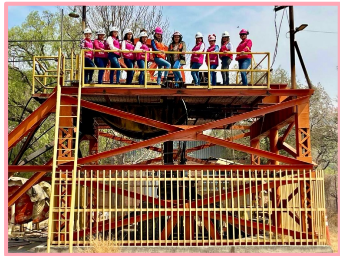
(The rehabilitated Cata Shaft with team members from VMC)
